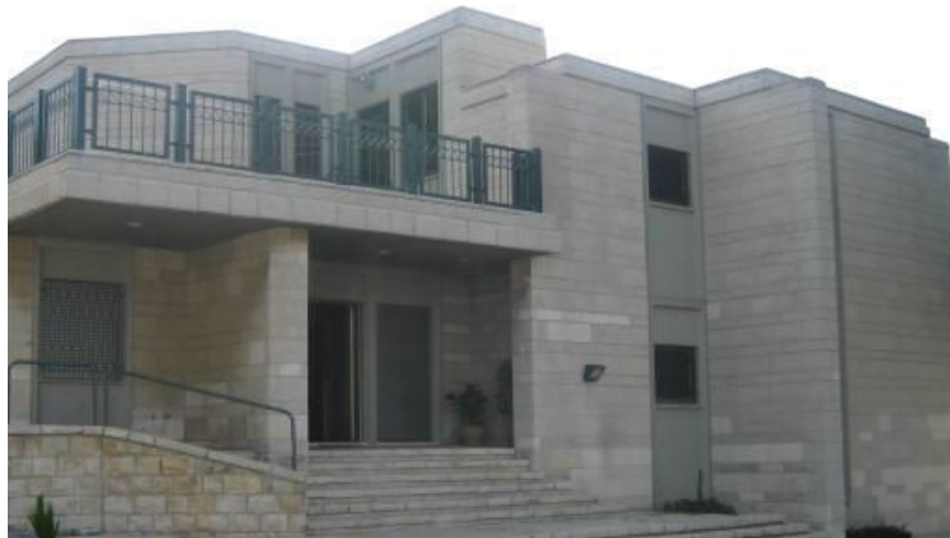
New Construction in Jerusalem.
